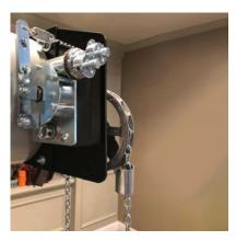
**GRIFCO HOIST:** Durable and reliable hoist for both normal operation and emergency descent of the door in case of fire.
